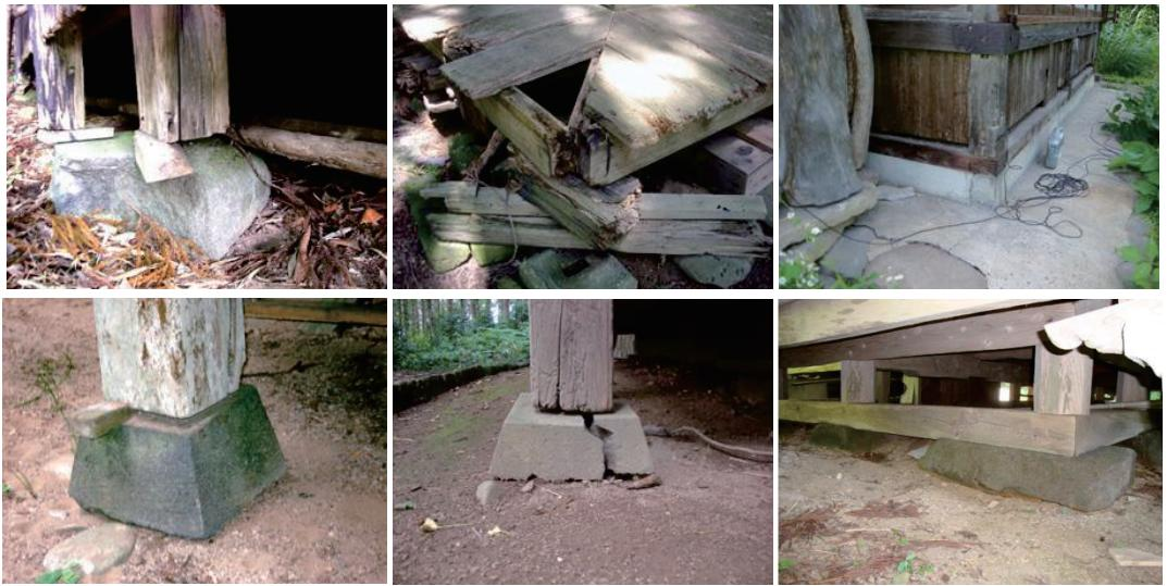
Fig. 2. Details of the damages at the bottom of columns
