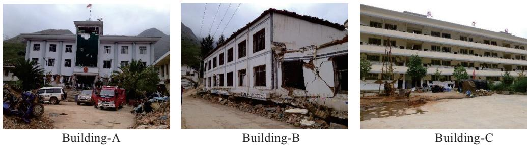
Photo 2. Typical damage of mutistory masonry buildings (locations are shown in Photo 1)
