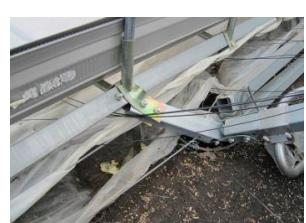
(f)柱・梁接合部の破断
