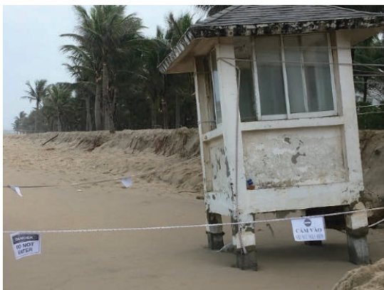
Figure 3. A corner of the guard house and fence of a resort were destroyed by waves (January 28 th , 2018)
