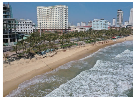
Figure 4. Erosion of My Khe beach (February 21 st , 2021)
